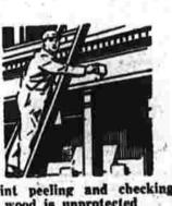
Paint peeling and checking so wood is unprotected
